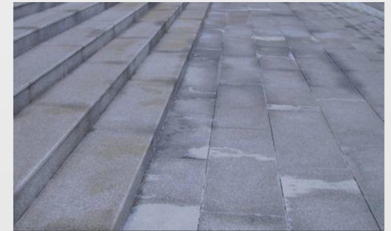
Efflorescence and whitening
