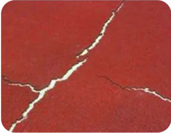
Runway cracking
