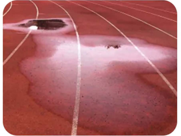
Water seepage and bubbling
